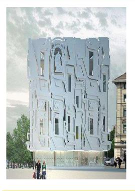
To ensure waterproofing and optimal conditions of humidity and temperature inside, a standard light skin that covers the machinery allows the use of vinyls for advertising purposes or for the visual integration in the environment.
