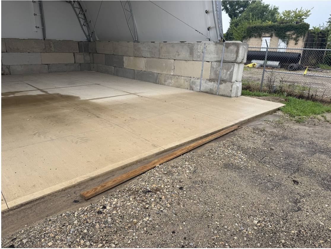
Figure A4. Adjacent slab / salt-barn-side condition requiring coordinated grading, drainage, and pavement transition work.
