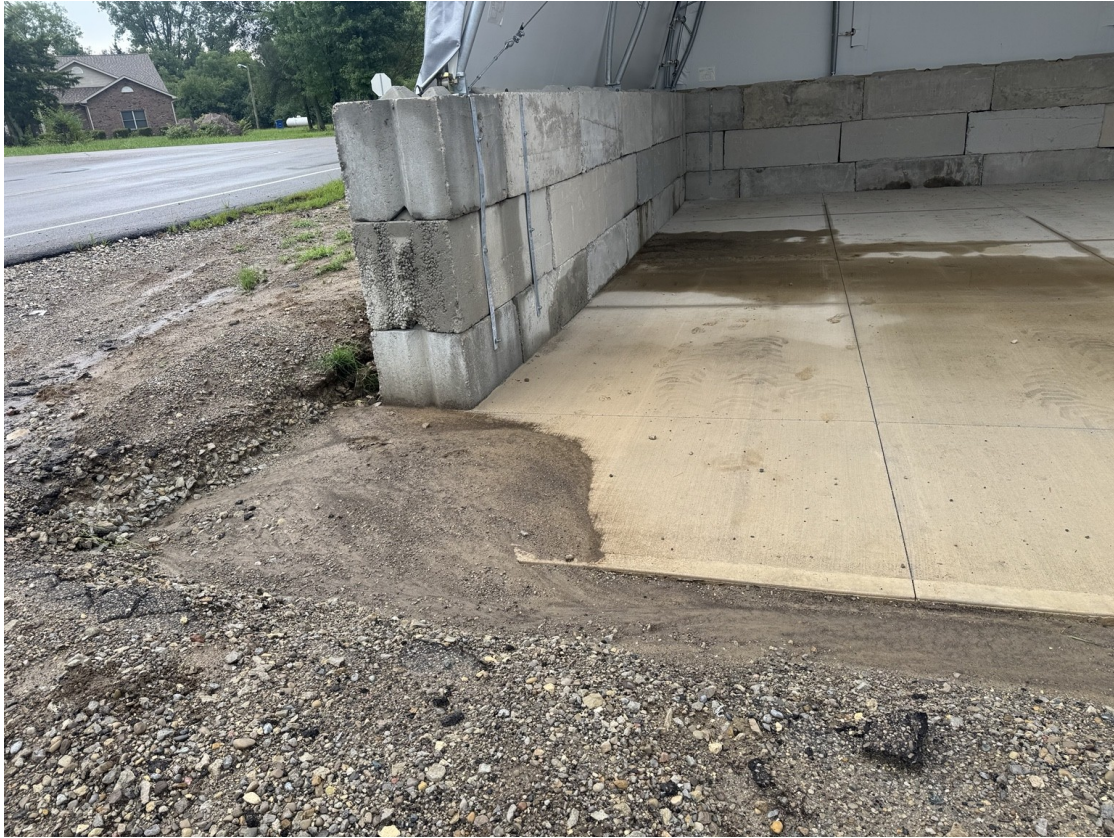
Figure A5. Additional slab / grade condition along the facility edge showing runoff and restoration considerations.
