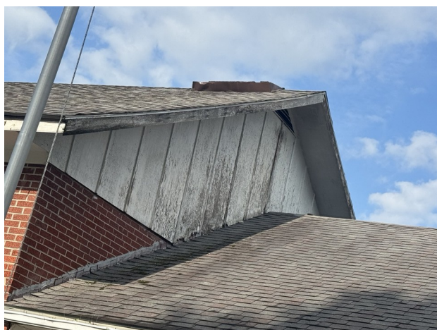
Figure 5. Roof-to-wall transition and existing flashing conditions.
