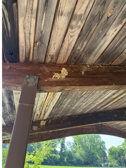
Figure 5. Wide underside view of the shelter roof structure, exposed wood beams, support post, and additional interior wood ceiling conditions.
