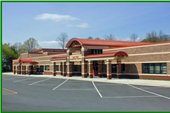
Rock View Elementary School 3901 Denfeld Avenue Kensington, MD 20895 Phone: 301-929-2002 Fax: 301-962-5986
