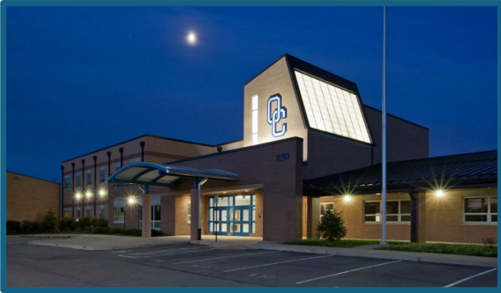
Oldham County High School
