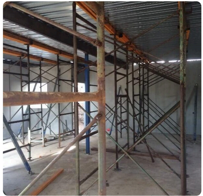
TRADITIONAL SLAB — BACK-PROPPED
