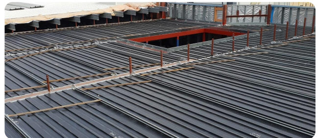
SPEEDFORM TRAY DURING INSTALL
