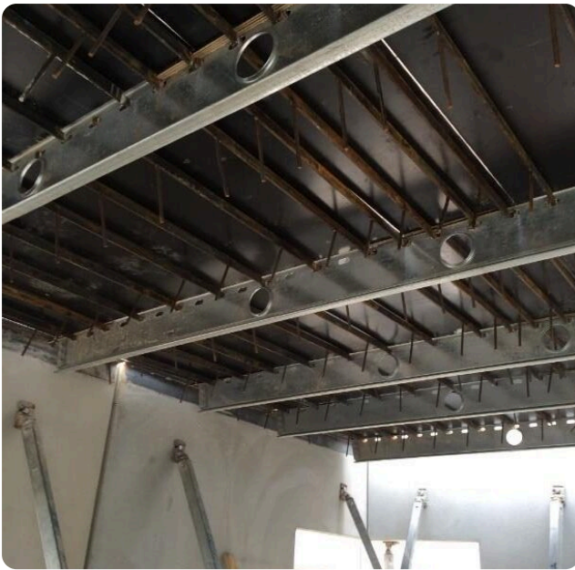
SPEEDFLOOR — NO BACK-PROPPING
