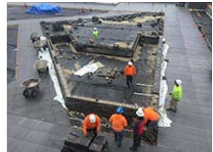
Allan Block Raised Planter Install
