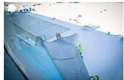
Waterproof Membrane Install
