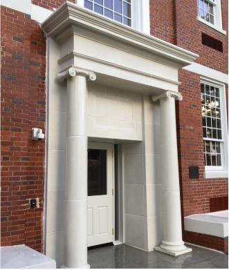
The craftsmanship involved made it possible to perfectly replicate the intricate woodwork from the original entryway but with a more durable material. Also, because it's lightweight, there was no need for the addition of costly structural steel.
