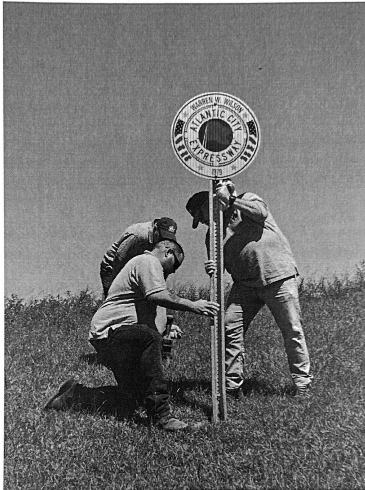
SJTA Operations crew install one of three memorial signs in honor of fellow workers killed on the job as highway workers [SJTA photo/Darleen Adamo]
