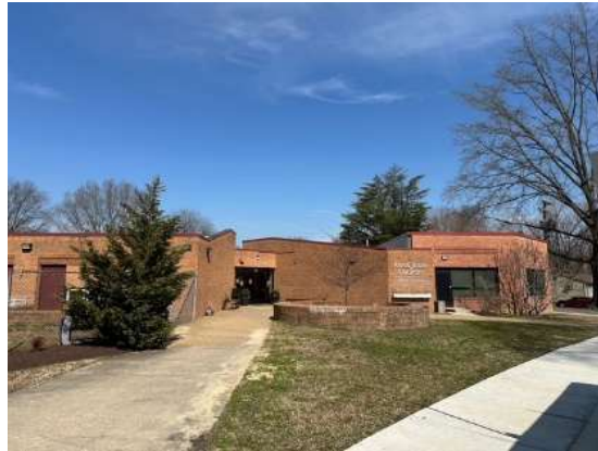
Anna Julia Cooper School (construction of new lower school, middle school, and current lower school)
