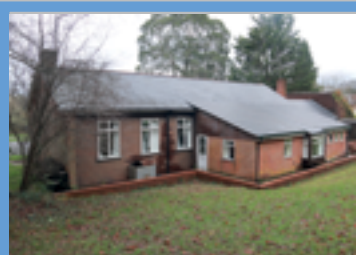
REAR OF THE BARN
