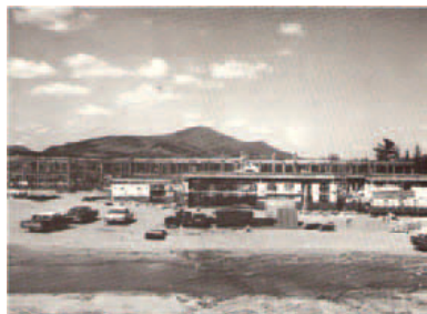
A view of the partially constructed Uihlein Mercy Center
