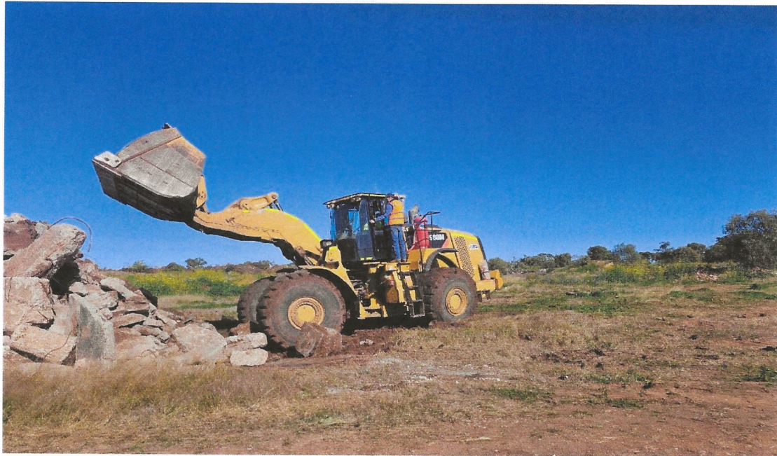
Plant operator training
