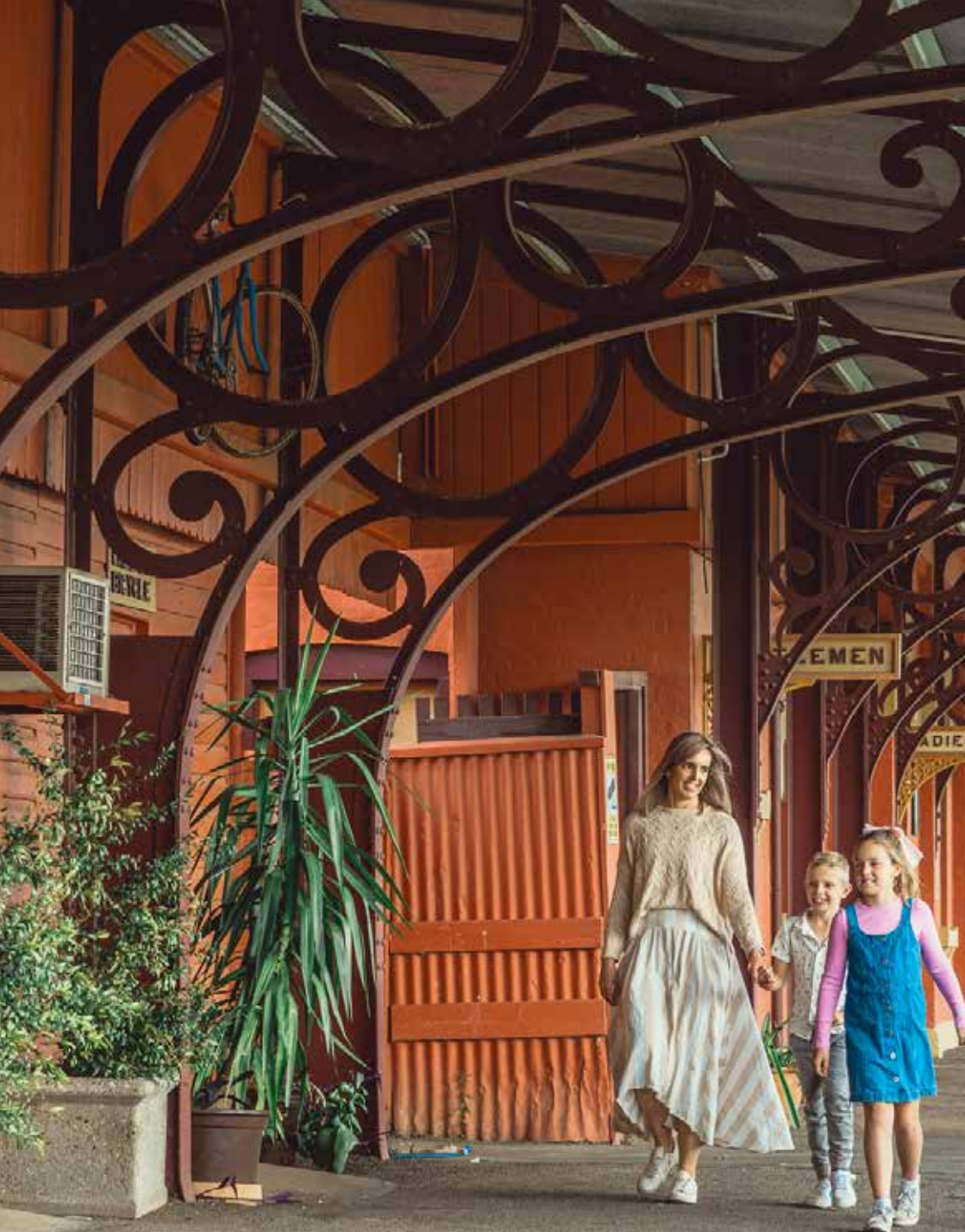
Pictured: Temora Railway Station
