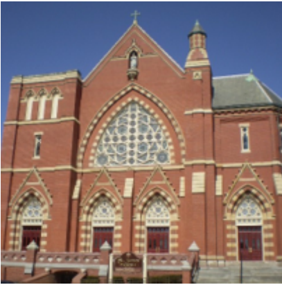
ST. JAMES CHURCH 185 WINTER STREET HAVERHILL, MA 01830
