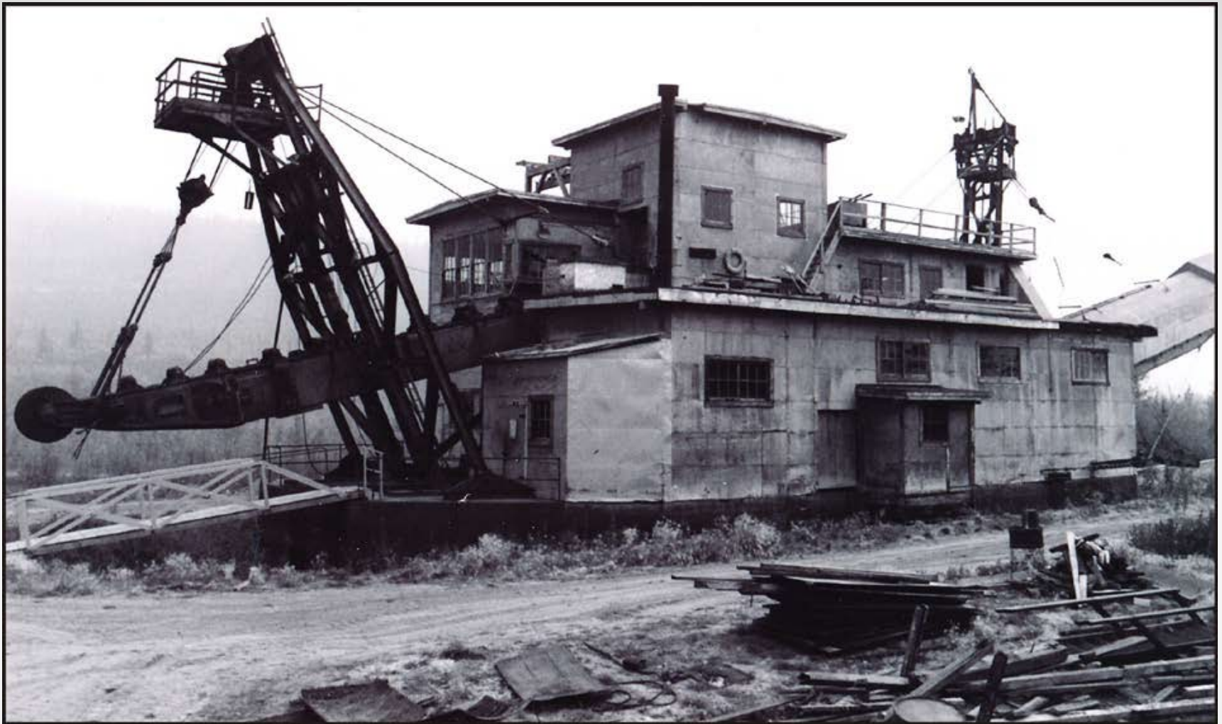
Dredge No. 4 at Chicken Creek, July 1975
