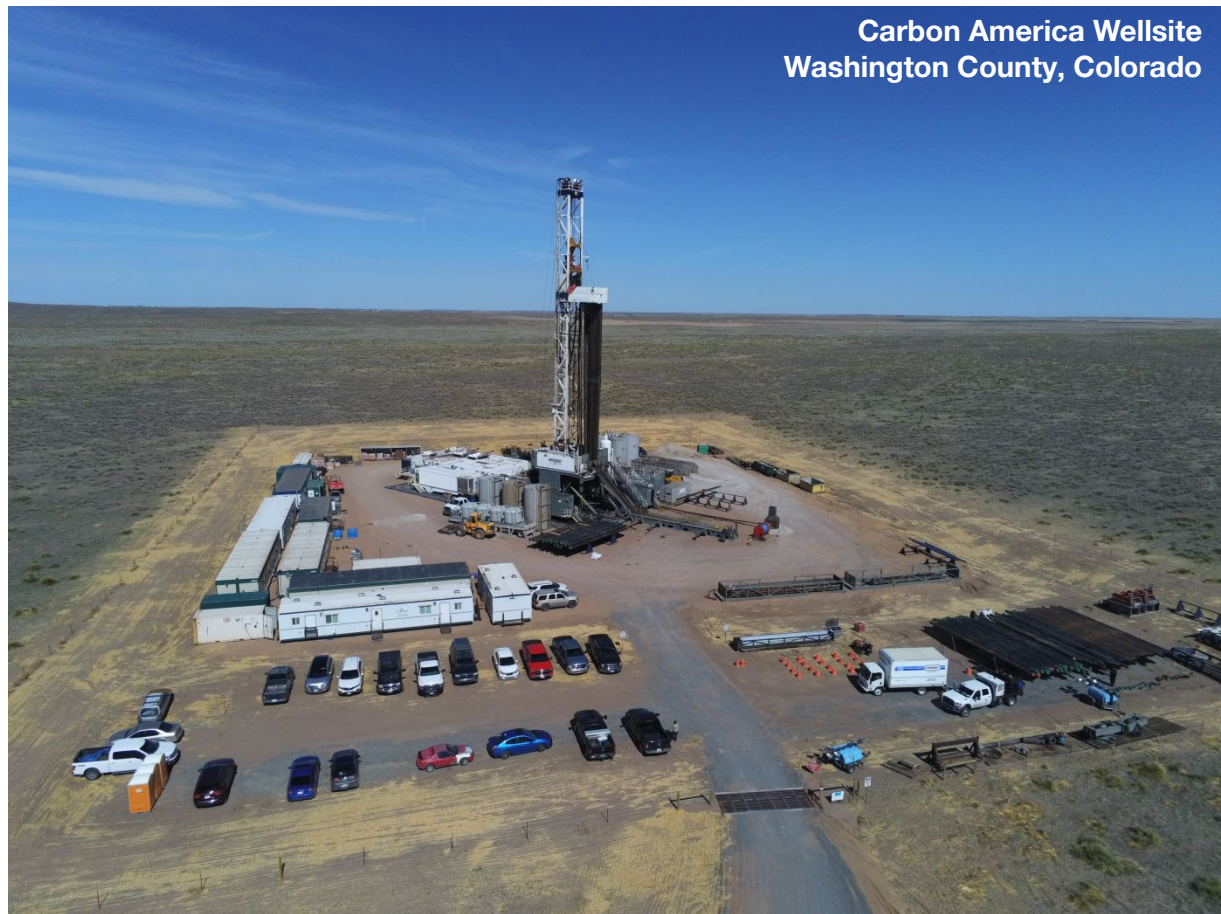
Drilling Operations (~5 weeks)
