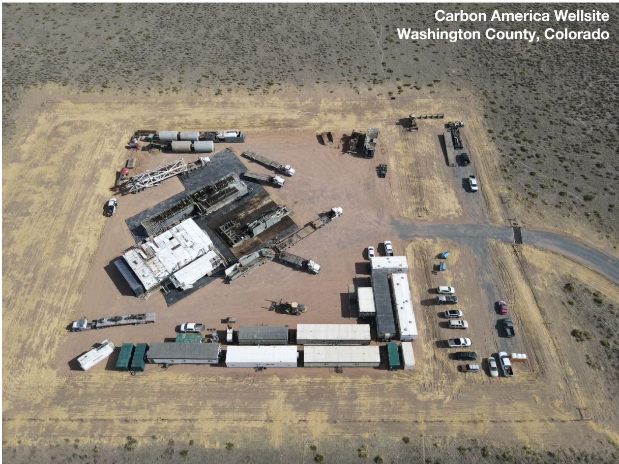
Wellsite Setup (~1 week)
