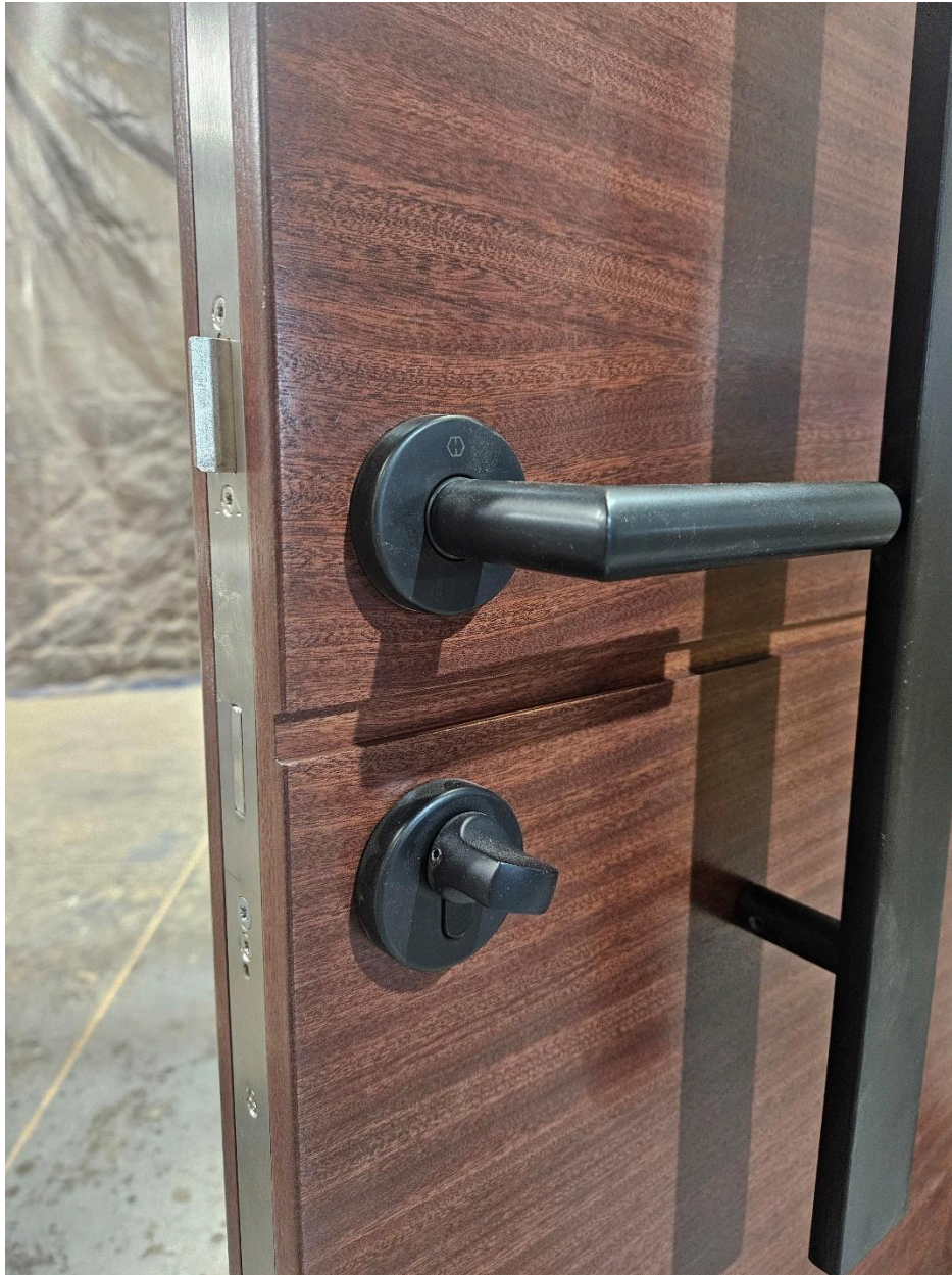
Thumb turn with lever added on interior
