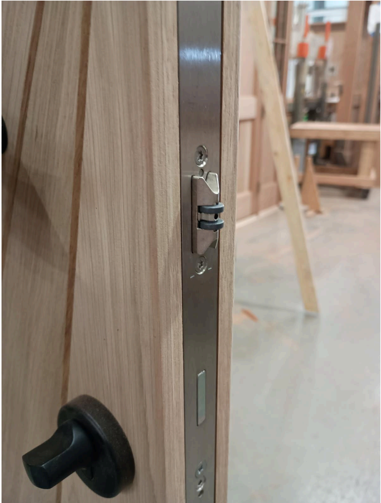
Roller latch installed
