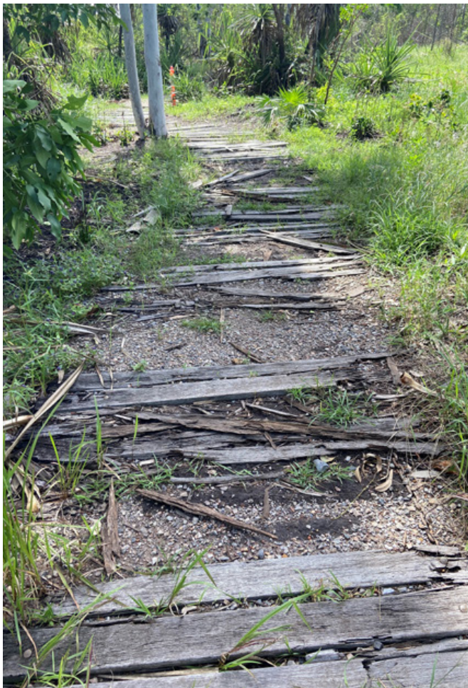
Figures 1 and 2: Reusing stockpiled gravel to cost-effectively repair an unsafe section of the Gurumbai Cultural Trail
