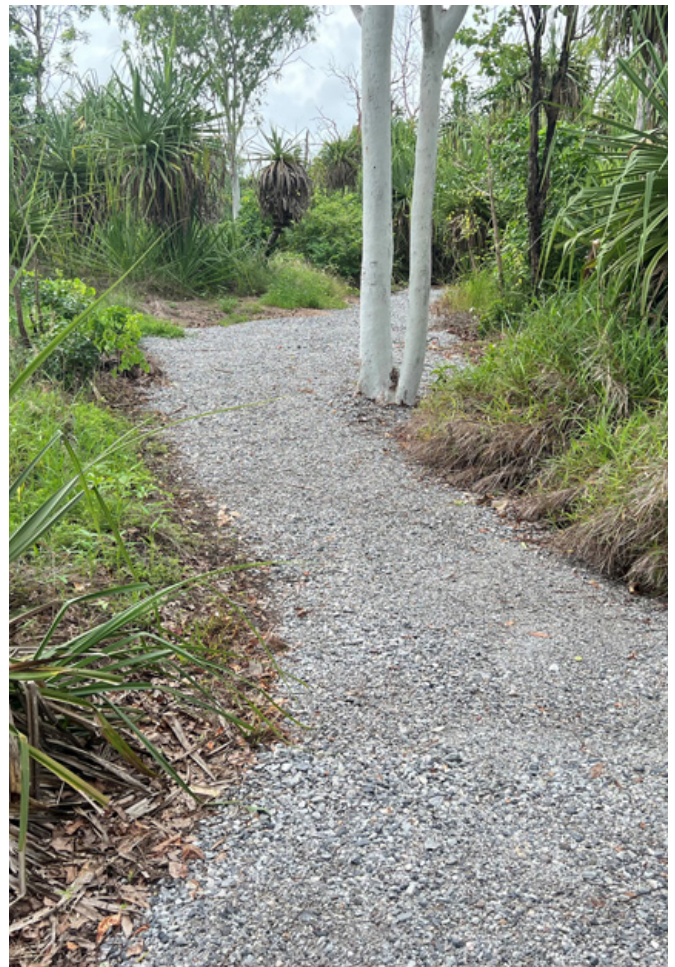
Figures 1 and 2: Reusing stockpiled gravel to cost-effectively repair an unsafe section of the Gurumbai Cultural Trail
