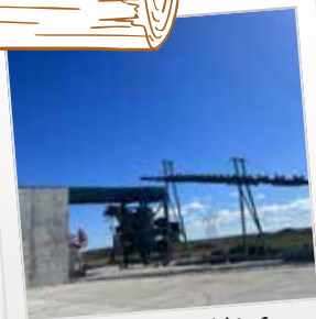
CONSTRUCTION OF THE NEW ROUNDWOOD MILL
