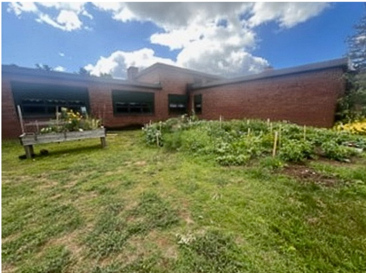
The garden area constructed at ExploreABILITY
