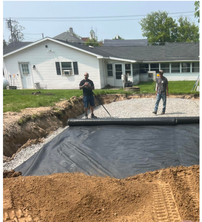
Outside of West Chazy during the septic tank replacement
