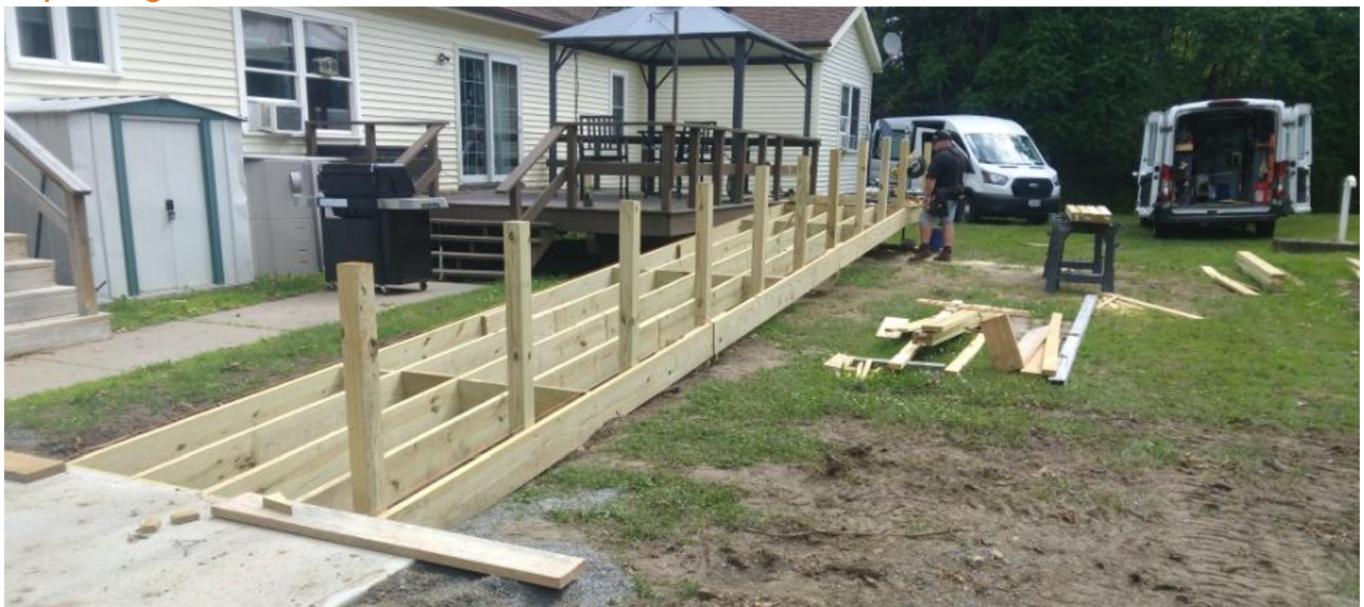
Replacing the boardwalk at the Salmon River Road IRA with a new concrete sidewalk
