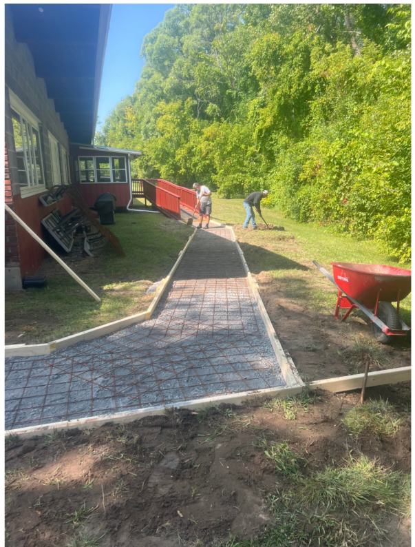
Progress as the team replaced the boardwalk at the Salmon River Road IRA
