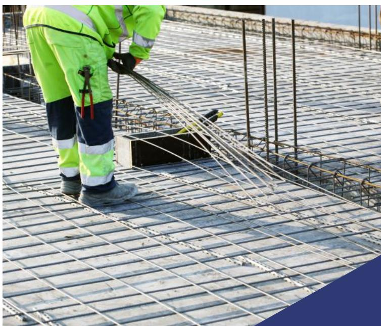
NJR Steel's reinforcing mesh is manufactured from hard-drawn wire and deformed cold-rolled wire with a minimum ultimate tensile strength of 510 MPa. It features a unique deformed wire pattern, known as the curry pattern, which facilitates superior bonding, stress-distribution and crack-width control.
