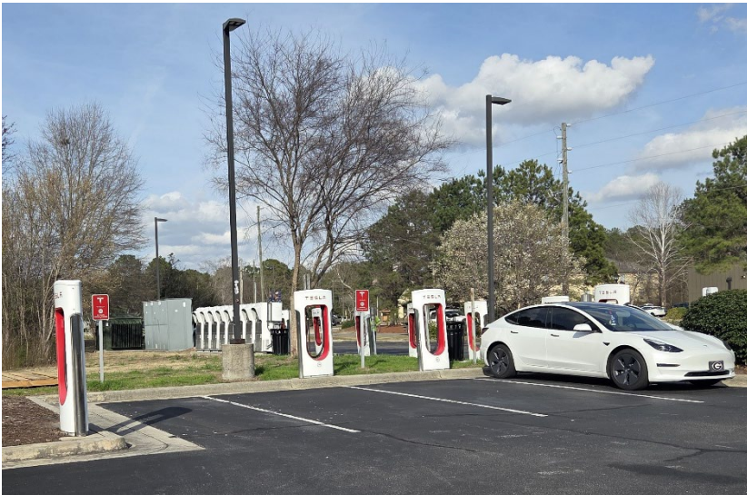
Interstate 95 Exit 49 Cedar Creek Road
