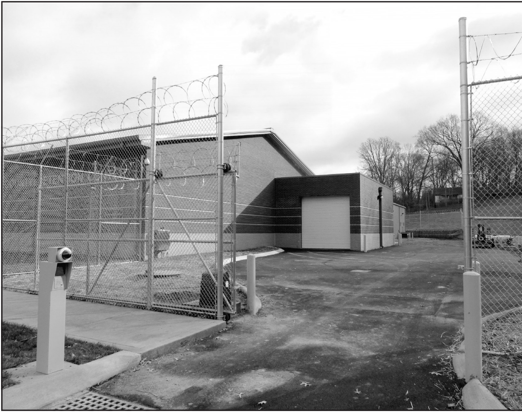
The high fence & security entrance is in place in front of the ‘Sally Port’ at the jail.
