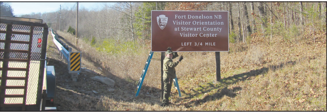
STAFF PHOTO Maintenance worker Ronnie Hicks works on getting new signs installed last Tuesday.
