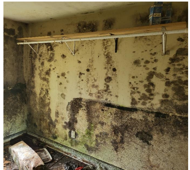
Figure 1-heavy mold basement drywall
