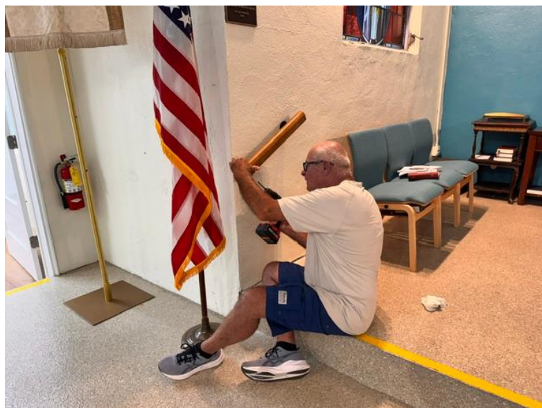
New Handrails Installed
