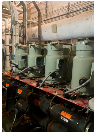
Demolition & Removal of Multistack module
