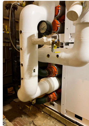
New Electrical, Insulation and Piping
