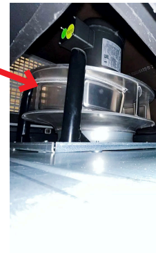
After Photos of DACD ECM Wind Wall Installed (shown is models 0734 and 2234 )
