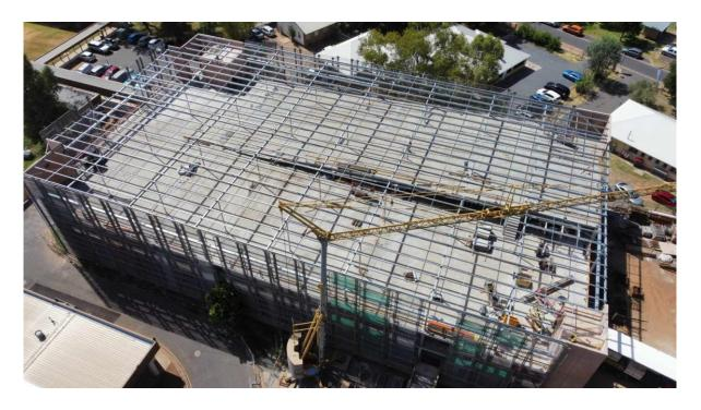
Under contract to Sunbuild Pty Ltd, the Alice Springs Multi Storey Carpark was a supply, fabrication of structural steel, delivery to site and onsite installation/erection project.
