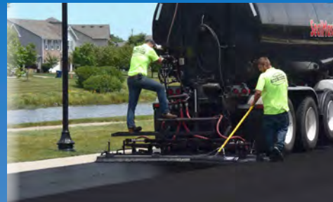
LIQUID ROAD SURFACE TREATMENT
