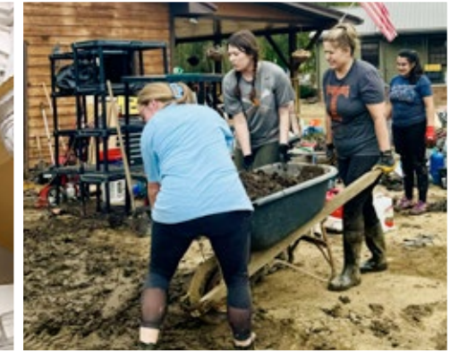
Telamon TN staff provide relief after Hurricane Helene devastated East Tennessee in 2024
