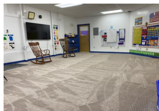
Freshly vacuumed carpet in the Pre-K classroom.
