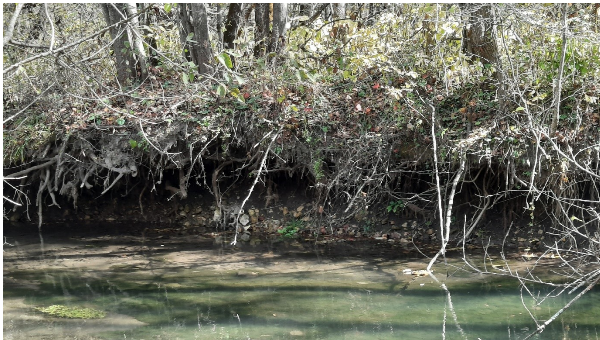
Image 8. Eroding stream banks in state forest land
