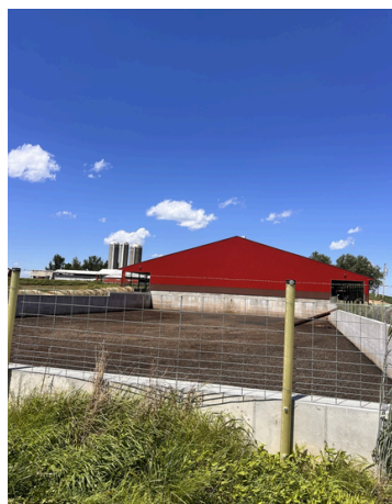
Manure Pit Completed in 2023
