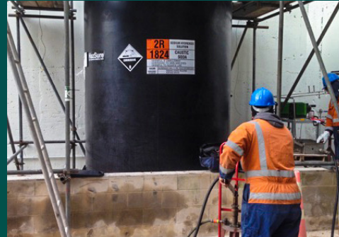
Ravensdown Tank Replacement
