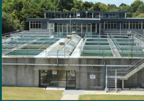
Hamilton City Council Water Treatment Plant Efficiency
