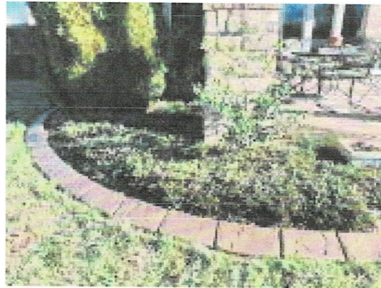
Continuous, Stamped Concrete Curbing
