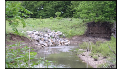
Streambank Stabilization Project
