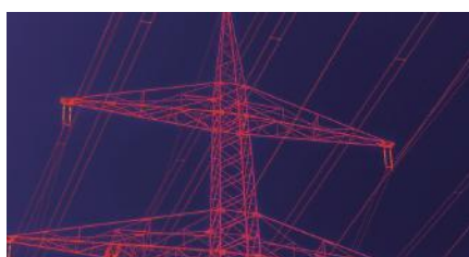
High-voltage Transmission Lines
