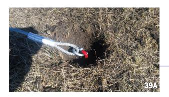
Anchoring cable and clevis connected to installed screw anchor. Soil type and elasticity data should be evaluated prior to determining screw anchor length and location.
