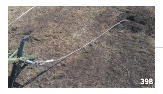
Anchoring cable attached to K-2300sd barrier and screw anchor. Shown with anchoring cable. The maximum distance from fixed anchor point to barrier end connection is 4 meters.
