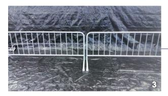
The ever popular pedestrian fence provides virtually no protection against a vehicle attack. While not designed to provide hostile vehicle mitigation many institutions only provide this kind of cursory protection.
