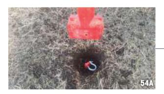
Screw anchor, subsurface, after installation, with screw type clevis affixed.
