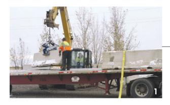
Concrete "jersey" or "diversity" barriers are impossible to move without heavy equipment, are slow to install, require multiple craft/trade groups, often slide on impact, are aesthetically unpleasing and obtrude the inbound/outbound operation of emergency vehicles.
