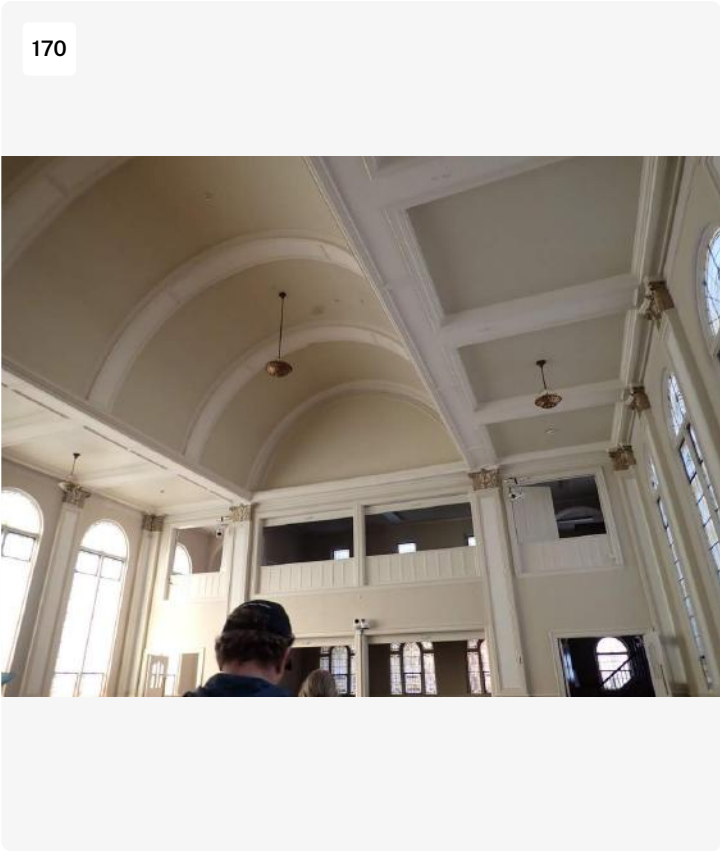
Project: Newnan Presbyterian Church Date: 11/9/2021, 9:25am
