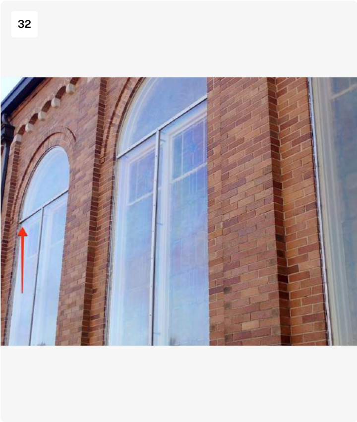
Displaced frame
