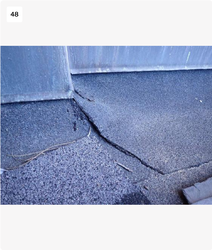
Minor uplift on lap seam
