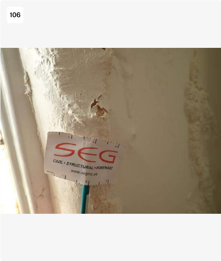
Efflorescence
