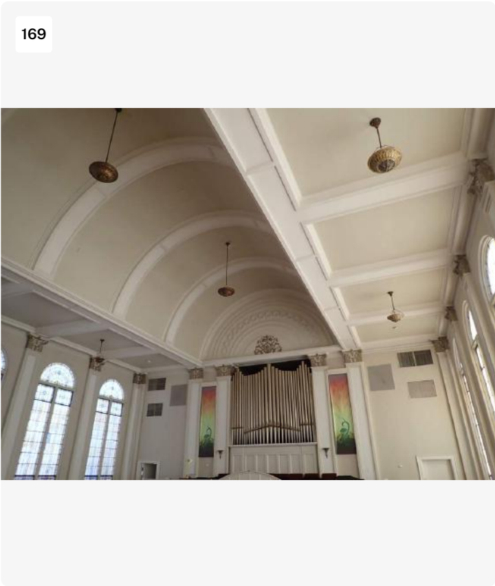
Project: Newnan Presbyterian Church Date: 11/9/2021, 9:52am
