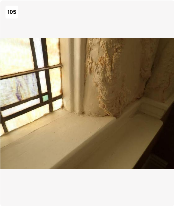
Efflorescence
