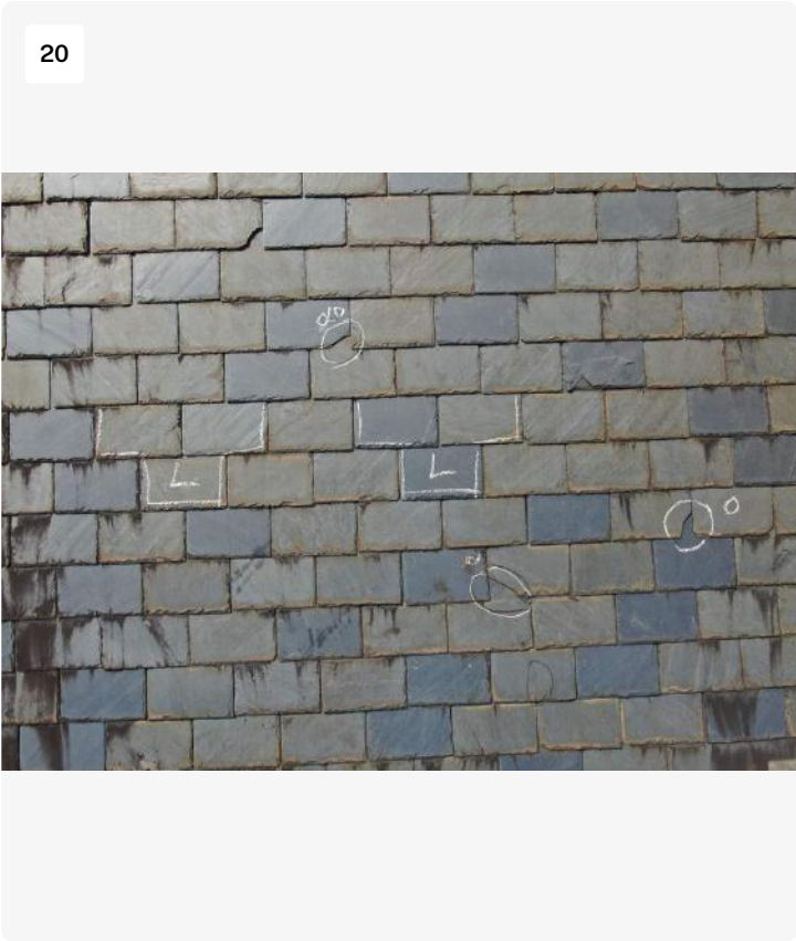
Old cracks were noted along with fresh cracks Displaced tiles
