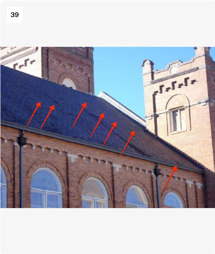
Displaced/missing tiles
