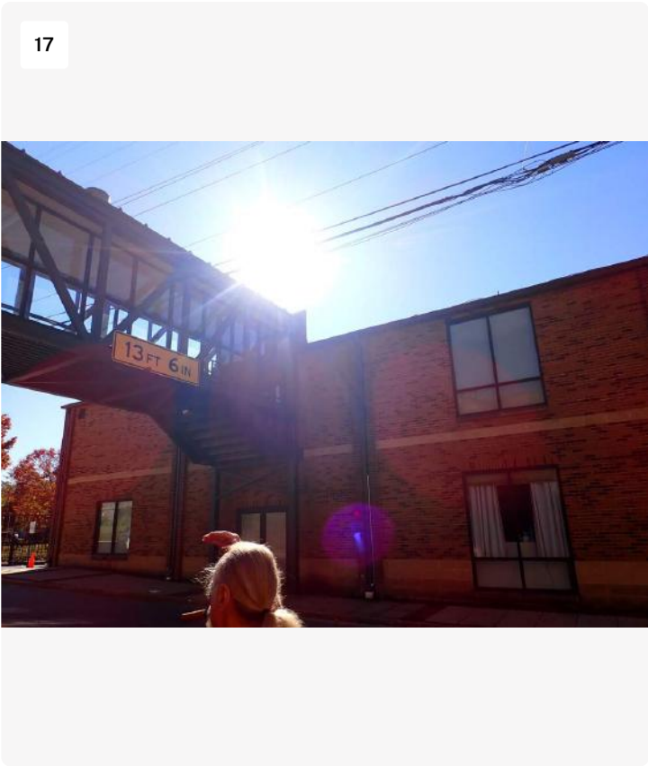
Building to the south of church
