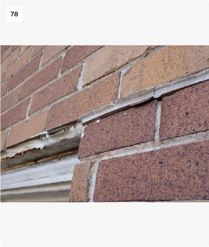
Displaced mortar
