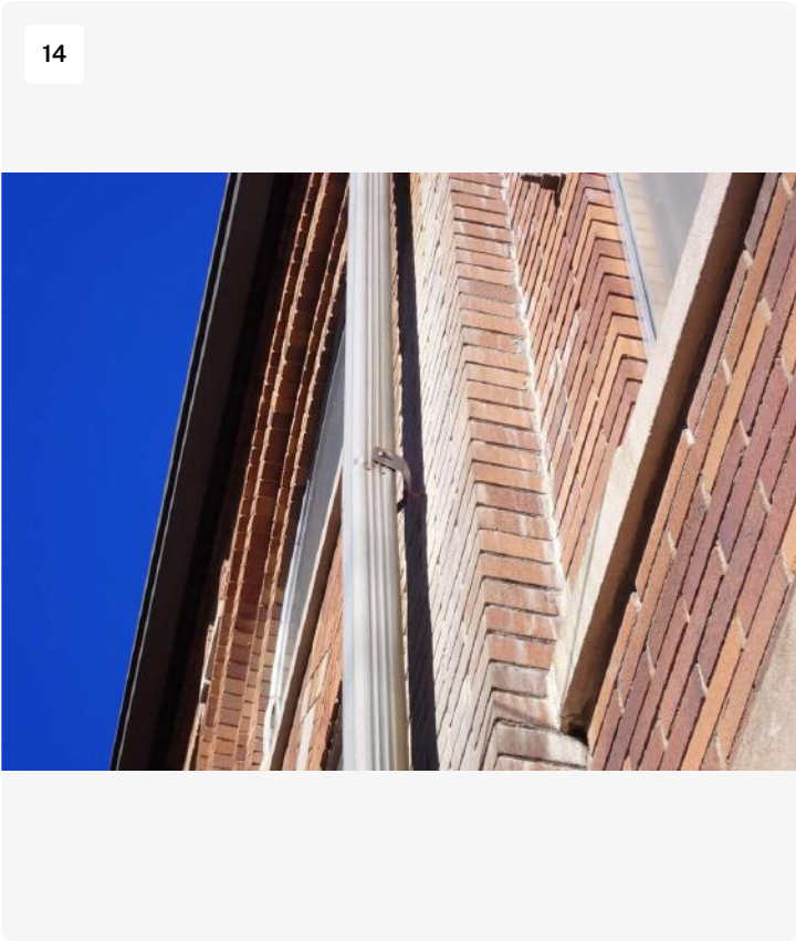
Displaced downspout
