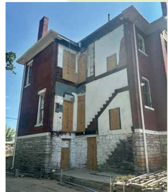
Below: Add-on removed as work begins to stabilize the foundation of our Victorian era house.
