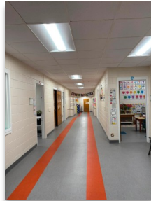
New ceiling, new lights, new energy!
