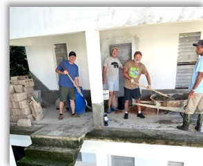
Concrete work in Cuba
