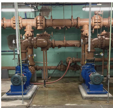
Photo (Above-left): Raw sewage pumps recently installed at the WPCP as part of Phase 1B. The project also includes new return pumps (photo above-right). This upgraded equipment handled an influent of nearly three times the average daily flow during heavy rains this spring. Finally, the photo on the bottom left illustrates the new boiler units installed.
