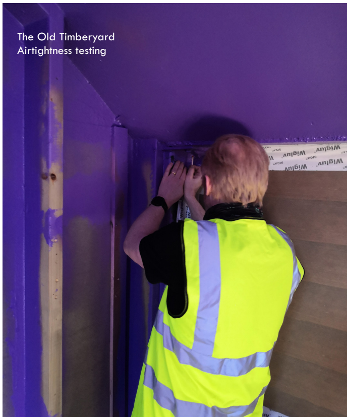
The Old Timberyard Airtightness Proofing, Using Passive Purple
