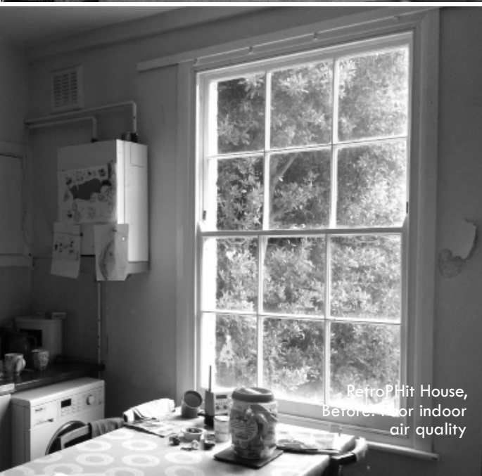
RetroPHit House Before
