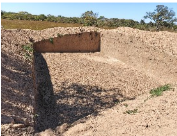
The reservoir ready to be lined and filled
