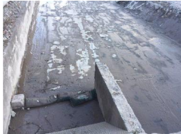
Stormwater Drain with filter near main gate
