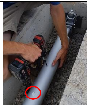
Drill and install extra feather clips if necessary
