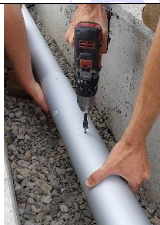
Secure tube joining screws
