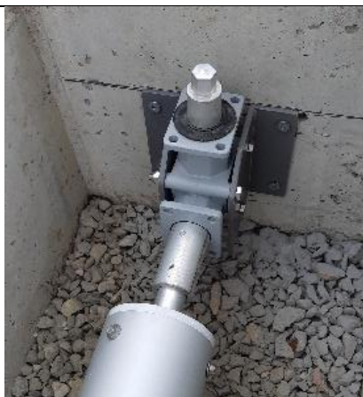
Insert tube assembly onto the end slug attached to the gearbox and screw in place
