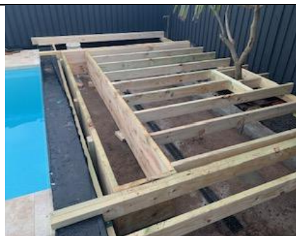
Cavity lining 190 x 35 or 245 x 35 as required
