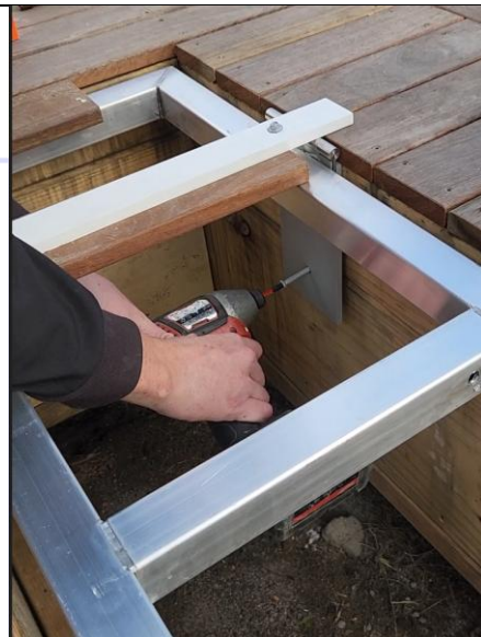
Predrill & screw bottom of Hinge Plate
