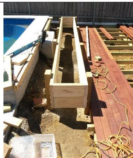
Cavity lining 190 x 35 or 245 x 35 as required
