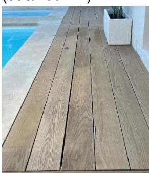
Millboard 176 x 32 (2 boards) Cut hinges into rear board
