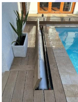
Millboard 176 x 32 (2 boards) Cut hinges into rear board
