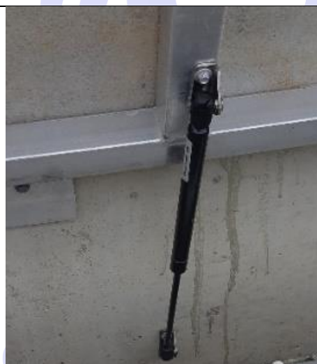
Completed Inside Strut
