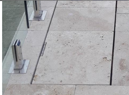
Cut tiles around hinges
