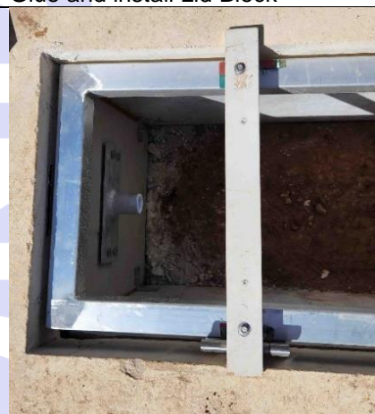
Support bracket ready for next hinge
