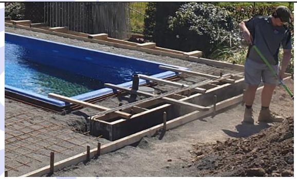
Pit formwork BRACED ready for concrete
