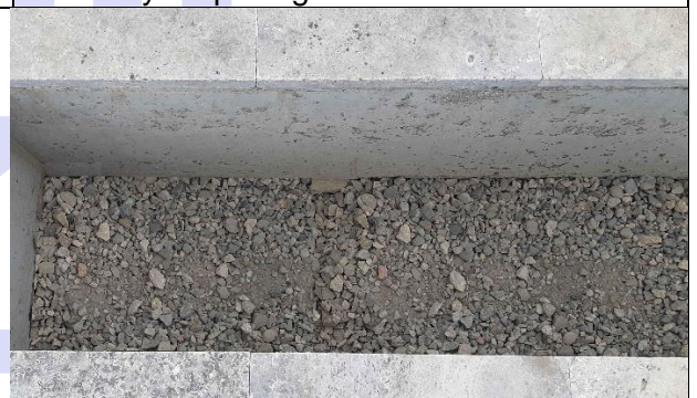
Gravel base with agi line underneath. Completed pit minimum 0.450m deep plus gravel and agi line.
