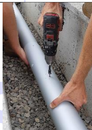
Secure tube joining screws
