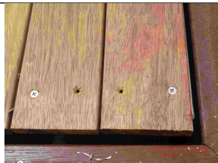
Pre-drill and countersink decking boards for lid
