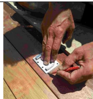
Marking handle position
