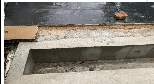
Completed pit with sloping concrete base and formal drain – ready for paving
