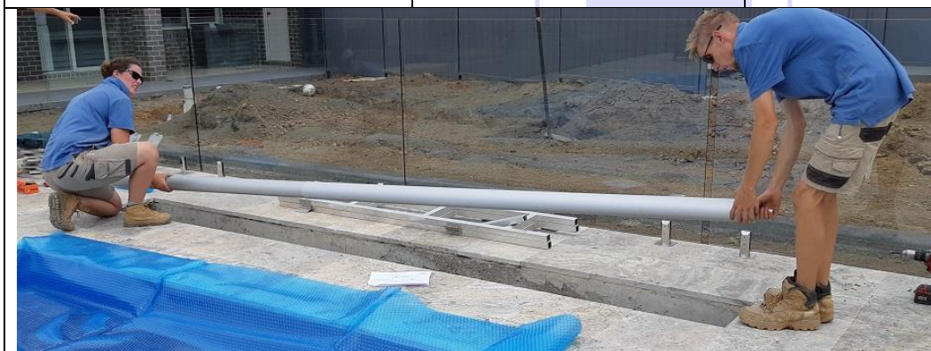
Insert the short End Slug into the End Mount
