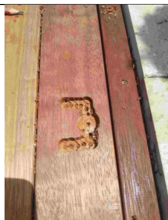
Completed drilling using speed bit
