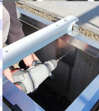
Predrill bottom of Hinge Plate
