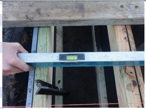
Figure 2 Ensure formwork is level horizontally and vertically
