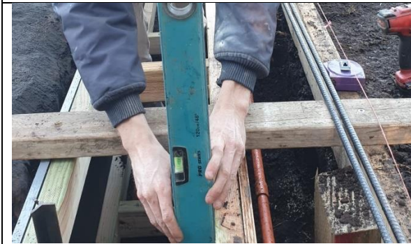
Figure 1 Form up concrete pit
