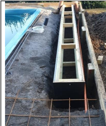
Figure 1 Form up concrete pit
